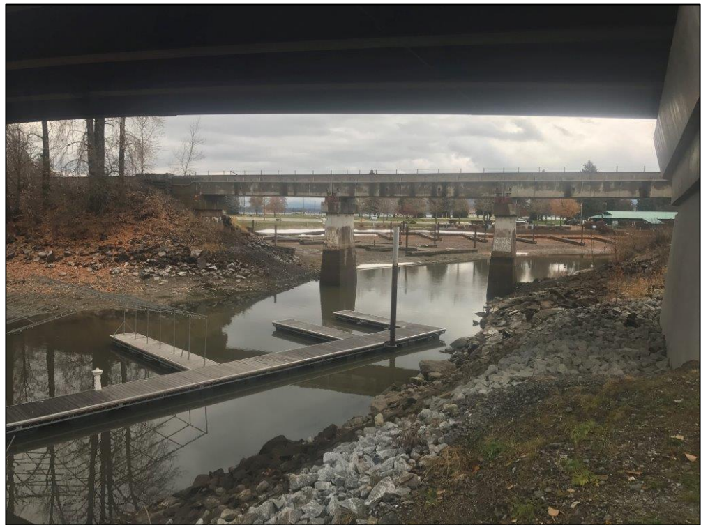
Figure 5. Winter elevation of existing Br 3.1, view downstream towards Lake Pend Oreille
